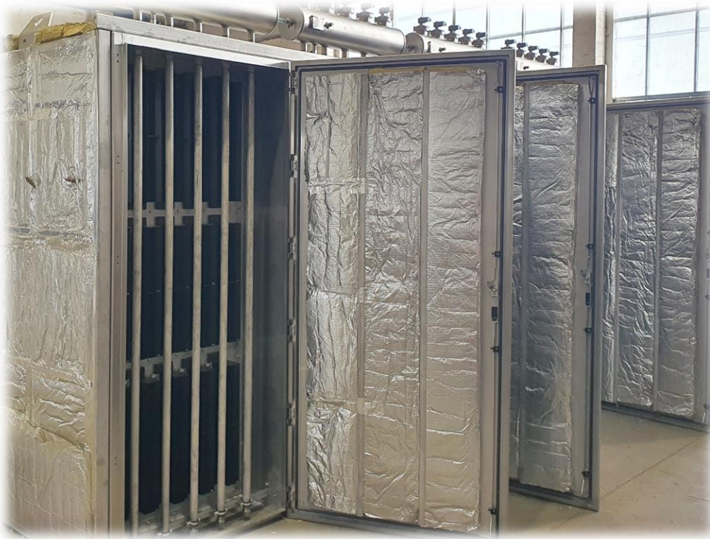
Before sheet metal cladding
